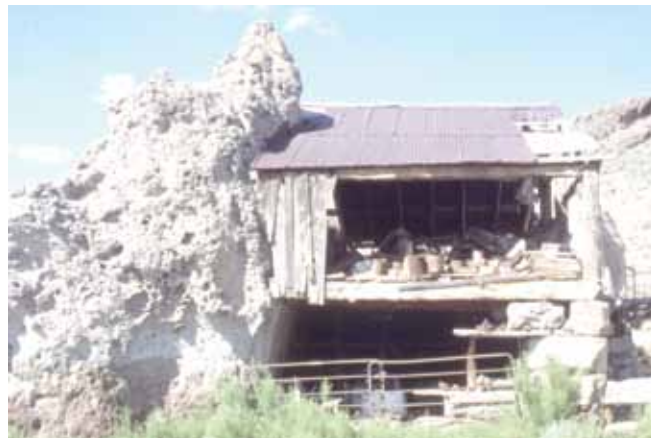
First barn built on Delmue ranch in 1880 is built against and into a volcanic stone outcropping.
