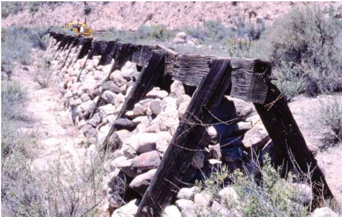
Water diversion dam built by Union Pacific in Rainbow Canyon.
